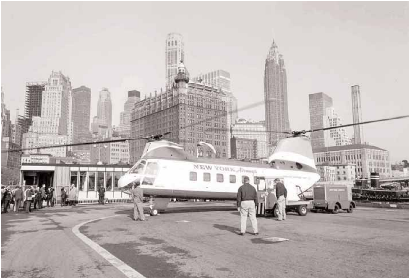
The facility was the first heliport in the United States to be certified for scheduled passenger helicopter service by the FAA.
